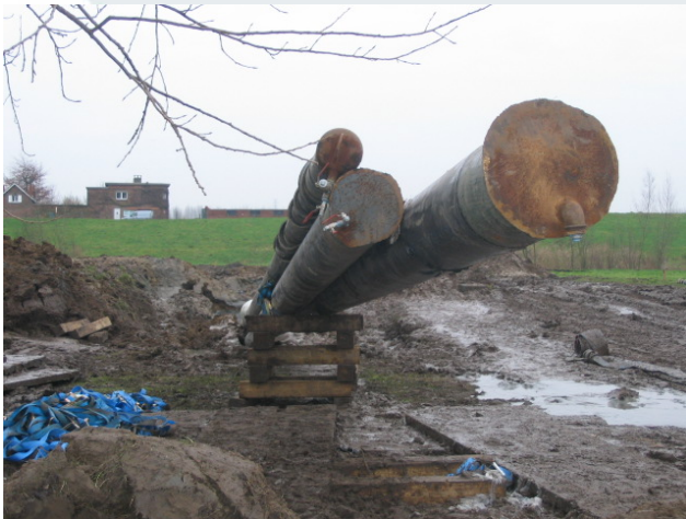
Directional drilling pipe string after pull in
