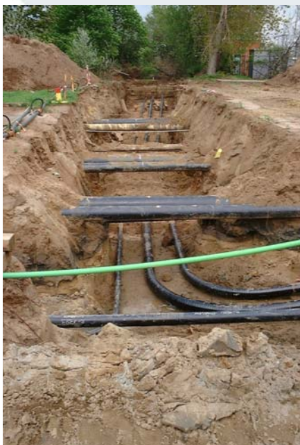
Pipelines crossing lines in pipeline corridor Scheldelaan
