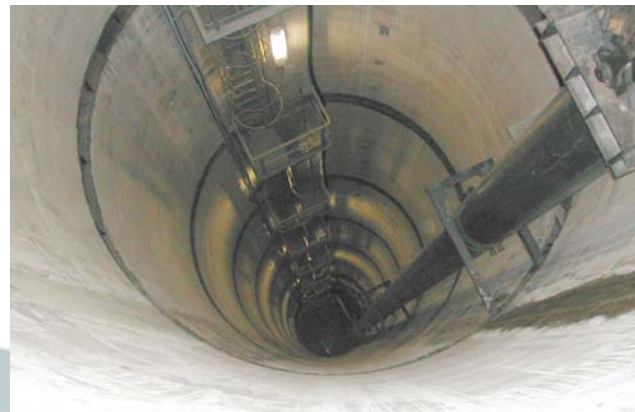
pipeline installation in shaft PALL-tunnel
