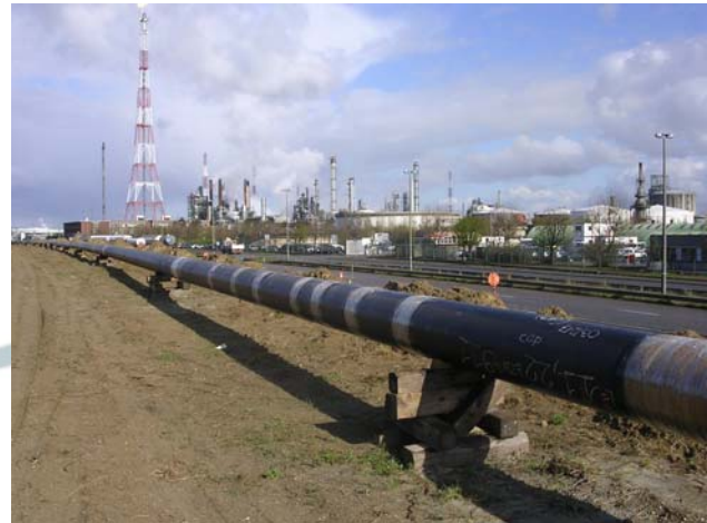
pipe strength preparation
