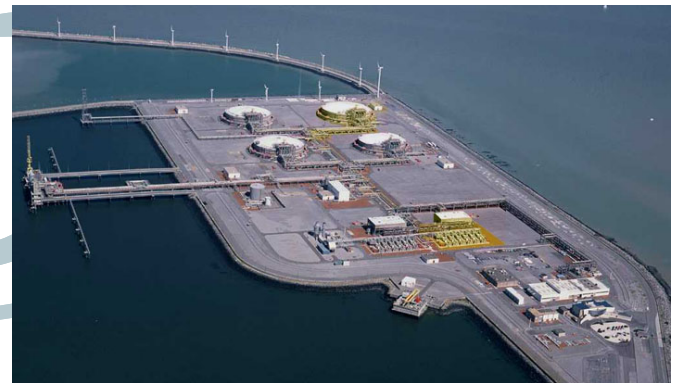
© Fluxys Infographics LNG terminal Zeebrugge - Extension works
