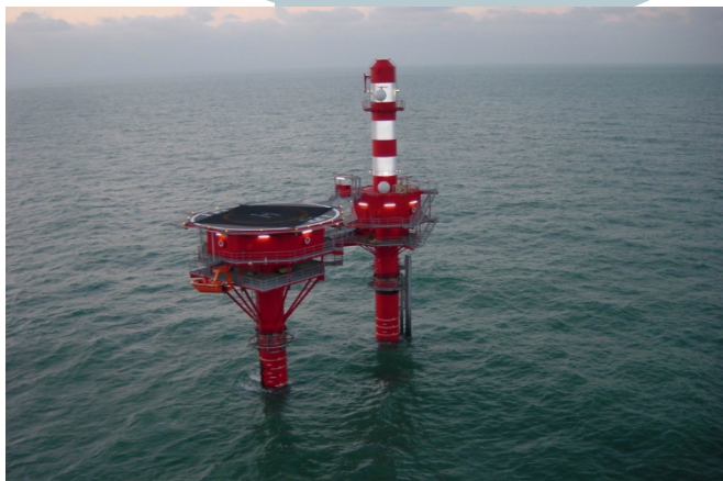
VTS radar station Oostdijckbank
