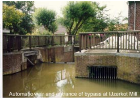
Automatic weir and entrance of bypass at IJzerkot Mill
