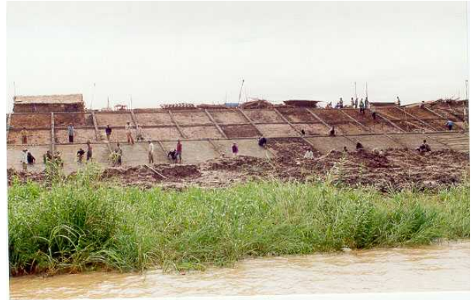
Bank protection works along the Tonle Sap Riverbank (Chaktomuk Junction)
