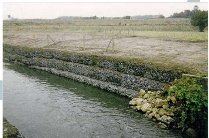
Riverbank protection (situation after works)
