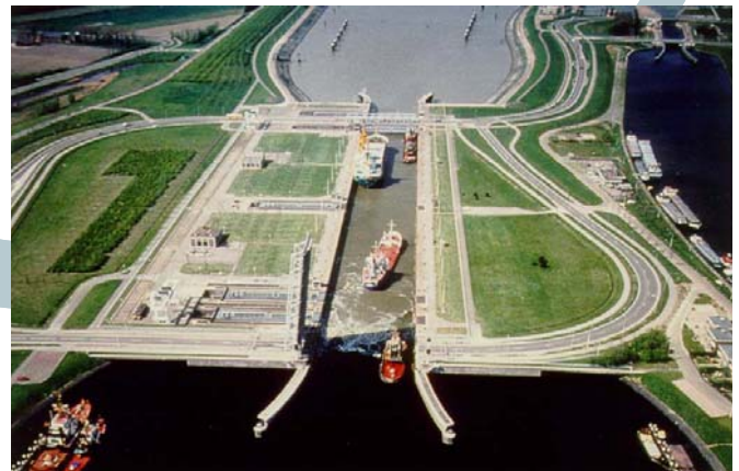
Terneuzen Lock Complex
