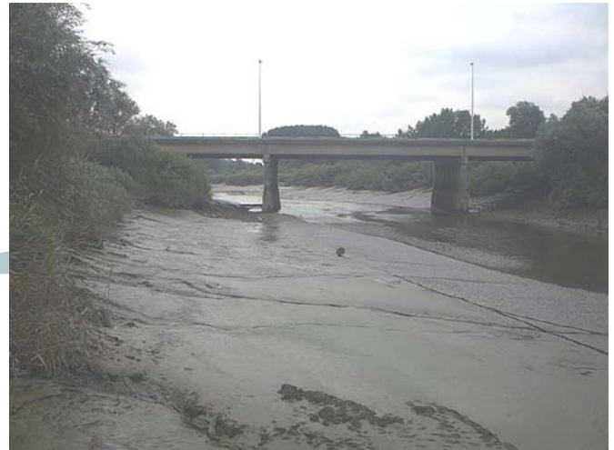
Sedimentation in the tidal Durme reach
