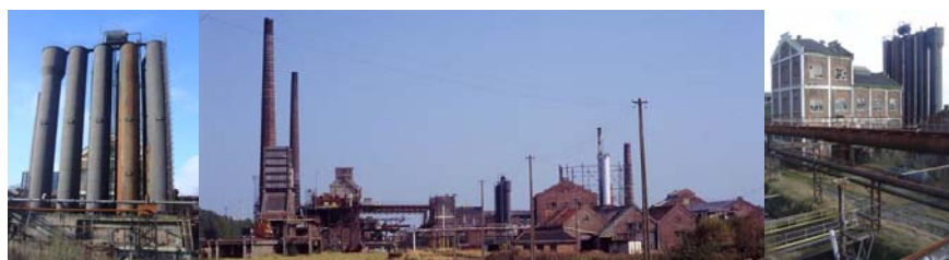
Figure 1. Carcoke before the remediation works (left: scrubbers, middle: general view, right: benzol factory)
